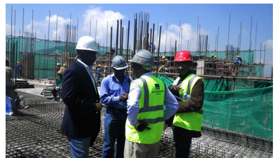
Life and fire safety auditing for IFC - funded project (Kigali, Rwanda)
